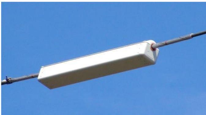
Bild 1: "Energieflusscontroller" – Distributed Series Reactor (DSR)
